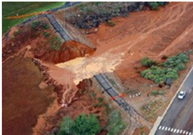
Figure 4-30 Laub Detention Dam Failure
